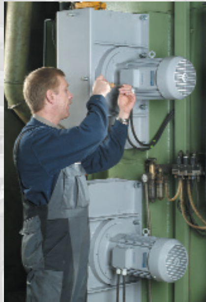
Used machines are technically overhauled and then integrated into plant operations. Working on its own or as a general contractor, AGTOS undertakes disassembly, transport and re-assembly of the machines.
