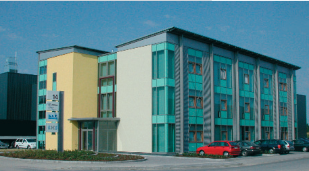
View of AGTOS' new head office in Emsdetten (Entry Mai 2003).
