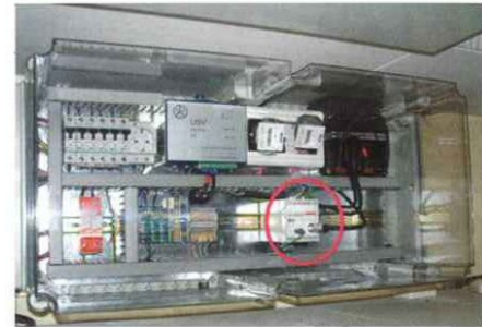
The radio telecontrol master is partly used as relay for substations far away
