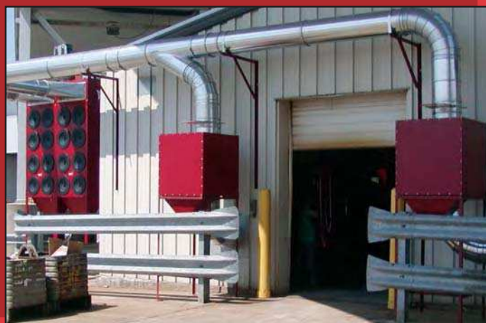
RP8-2 with spark arrestors collects laser smoke.
